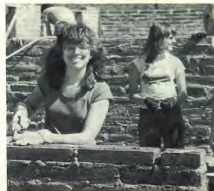
UCA seniors Laura McGlothlen and Lynette Kites laying bricks on the new boys' dormitory at Tesopaco, Mexico.
