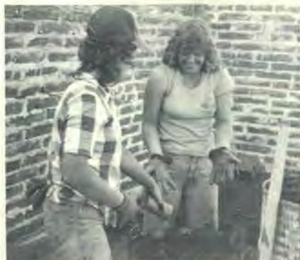
UCA seniors Judy Cunningham and Kim Kraft soak bricks before they are laid on the new boys' dormitory at Tesopaco, Mexico.
