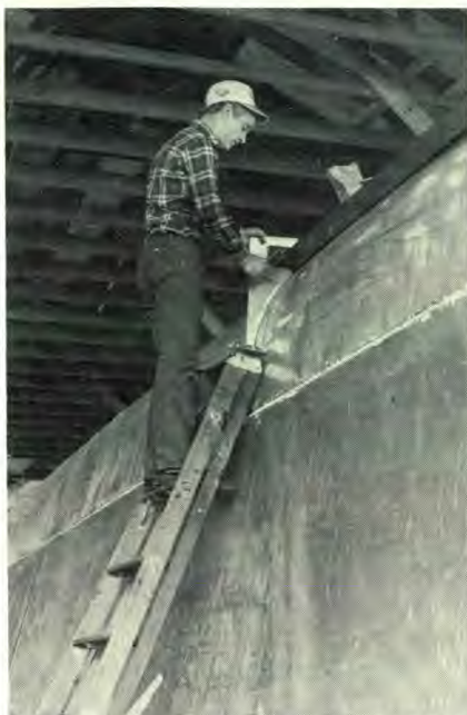
Volunteer Leroy Frederickson, an electrical and mechanical technician, builds a support frame which helps in moving the ship's hull.
