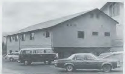
This recently completed addition to the Medford Church houses the Community Services Center on the lower floor and the Fireside Room on the upper floor, which is used for outreach programs of the church.
