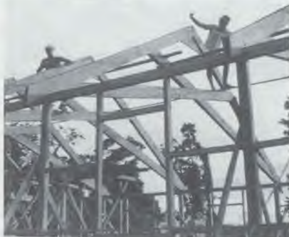
Students erect the roof trusses for the new church.
