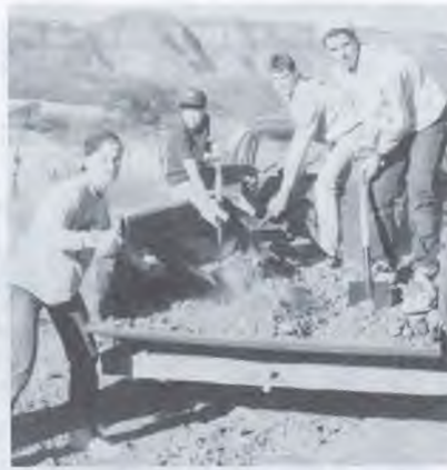
From the left, Matt Powell, Mark Easley, Jeremy Douglas, and Justin Still shovel gravel from a pickup truck onto the runway in the village of Nostic in Mexico.
