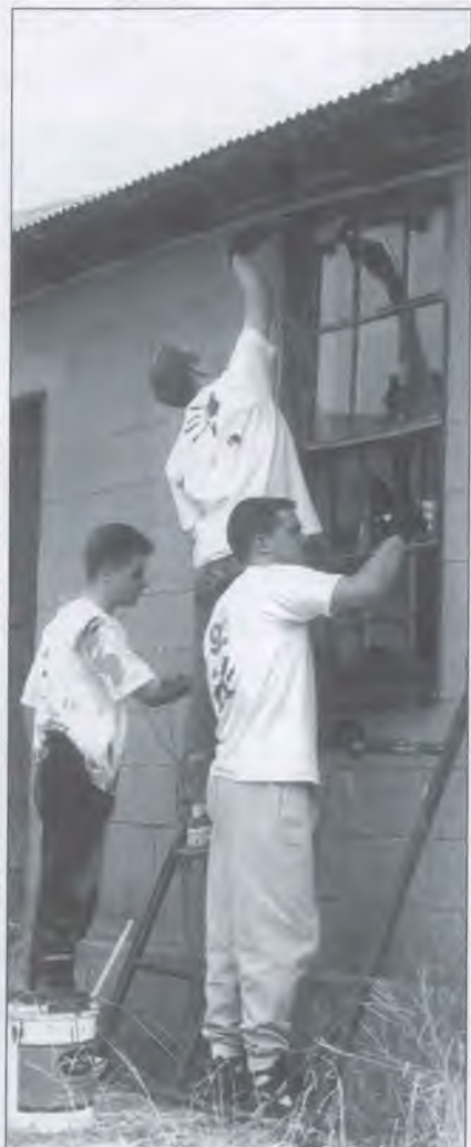
Seniors Ryan Dye, James Culmore and Matt Walsh apply exterior paint during the renovation of one of the Holbrook School buildings.
