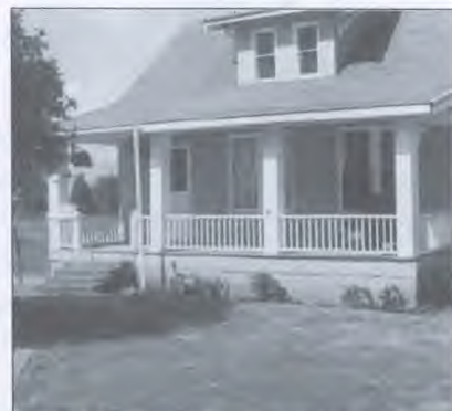
The 100-year-old home after camp meeting youths completed their renovation work valued at $4,000
