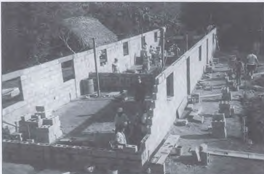
The walls of a three-room school go up in the remote village of Xalaquim during a visit by Gem State Adventist Academy volunteer builders, March 16-25.
