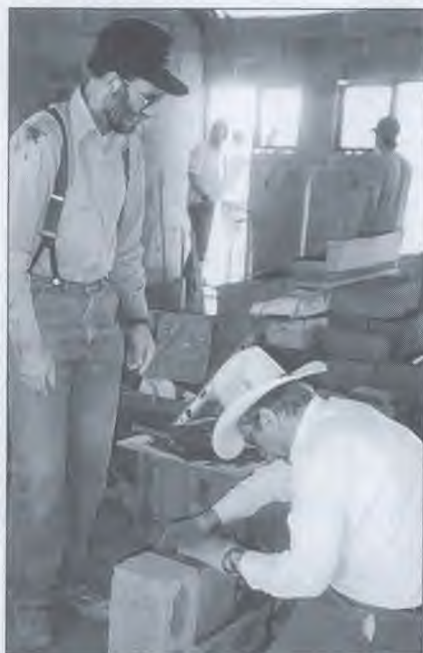
Phil Becker, left, volunteer leader of the group of builders from Lewis County, helps coordinate placement of interior walls as Harley Miller, M.D., constructs the cinder block wall partitions.
