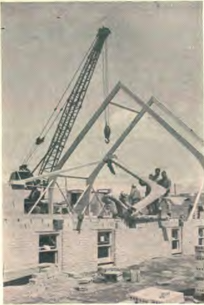
Workmen placing the large laminated roof arches in place.
