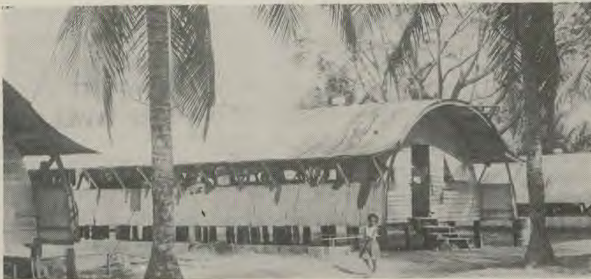
Worn out dormitories at Betikama Central School, Solomon Islands, soon to be replaced.
