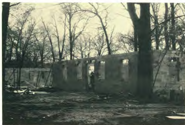
A view of the two cottages as they appeared on May 9, after 5 days of construction.
