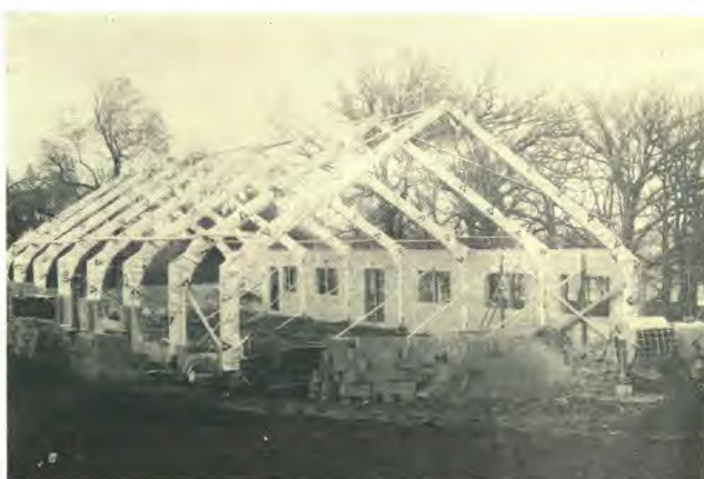
Building progress on the lodge hall as viewed May 9. Another two weeks and it will look quite complete.
