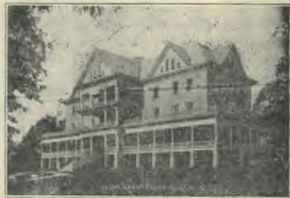
IOWA SANITARIUM, NEVADA, IOWA.
