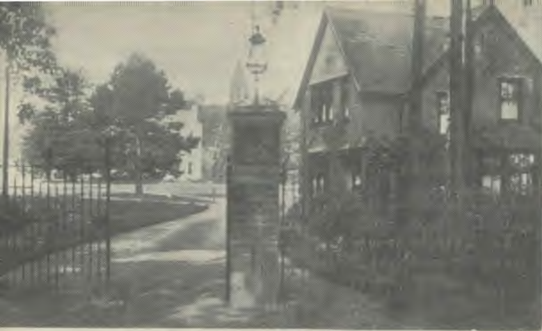
Entrance Gate, The Stanboroughs
