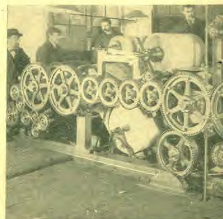
A printing press at Messrs Cassells which prints 10,000 lines per hour, registering the number printed.
