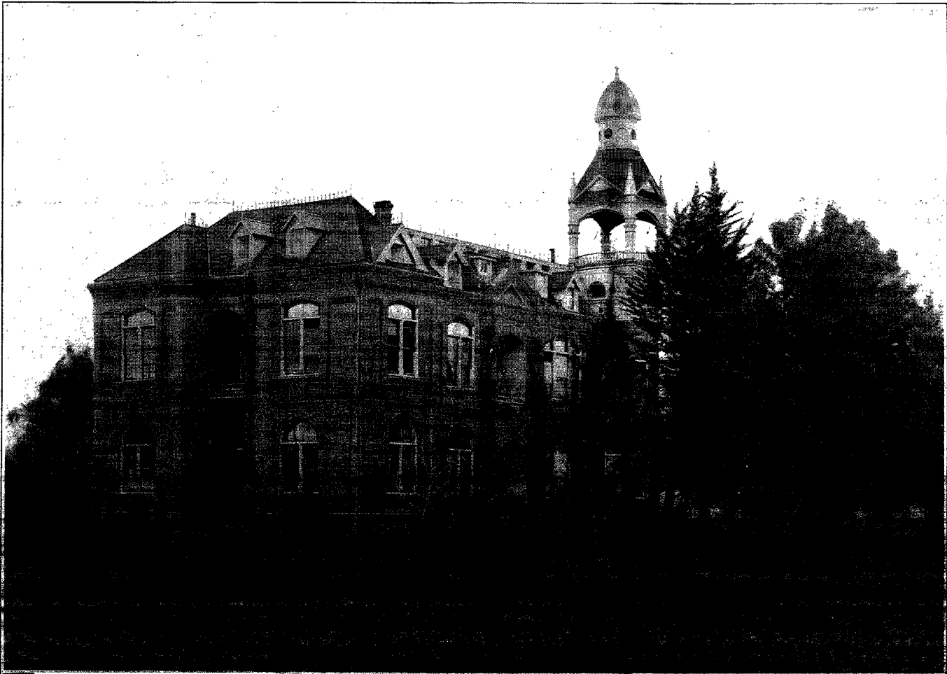
Fernando Academy, Main Building, Side View
