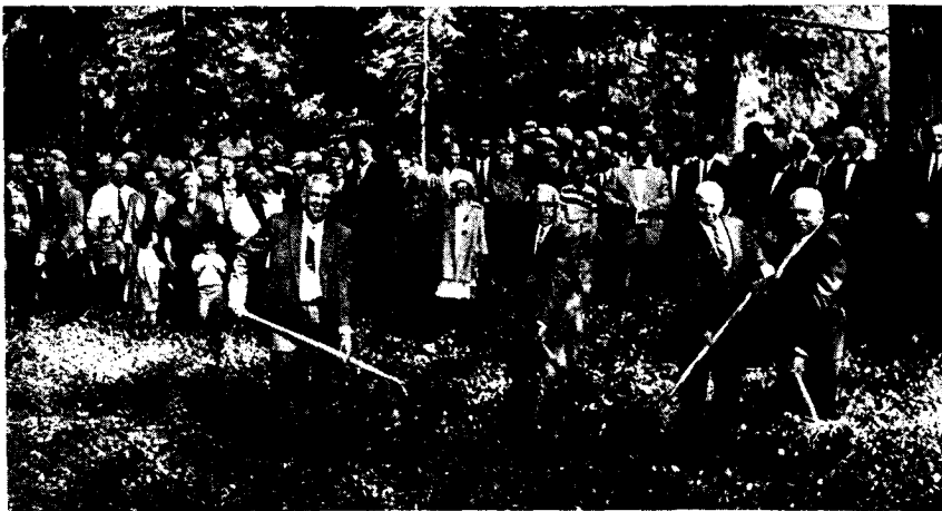
Ground-breaking ceremonies for the St. Helena church were held on April 22 with more than 150 people in attendance. Wielding the shovels are Elder S. T. Borg, pastor of the St. Helena church, Elder J. I. Robison, Harley Morrison, and Lloyd Landis. Brother Landis designed the building and will also superintend the construction. Others on the program were Horace Jenkins, Paul R. Alexander, Elder H. M. Blunden who told of the "Expanding Work of Seventh-day Adventists," and Dr. John E. Weaver who answered the question "Why Churches?" A trumpet trio furnished the music. The beautiful property for the church is located on Main Street. There is a little less than two acres in the plot, making it possible to have complete off-street parking. S. T. Borg, Pastor.
