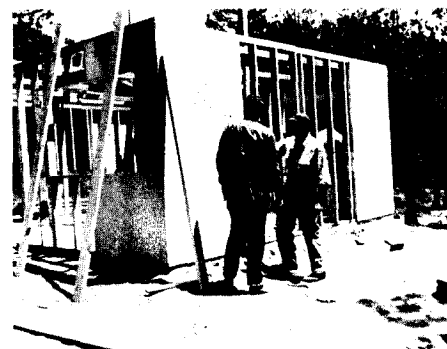
Brother Ray Hobson (right) is shown directing the construction of the ranch cabins. Brother Hobson and Carrall Davis from the Vista church acted as general supervisors for the cabin construction.
