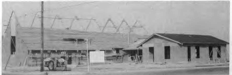
Rolinda church under construction.
