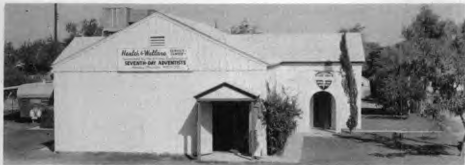
The new Health and Welfare service center located at 1426 East Maricopa Freeway, Phoenix. The building also serves as a storage department for clothing in case of a disaster in Arizona. Brother and Sister Kramer live in a trailer next to the building and are in charge of the center.
