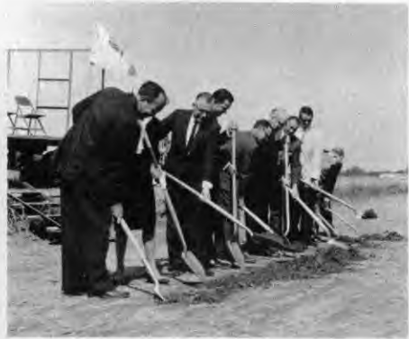
Gold-painted shovels were used at ground-breaking services by church officials and community leaders on Sunday, October 6, at the building site of the new Hanford Community Hospital.
