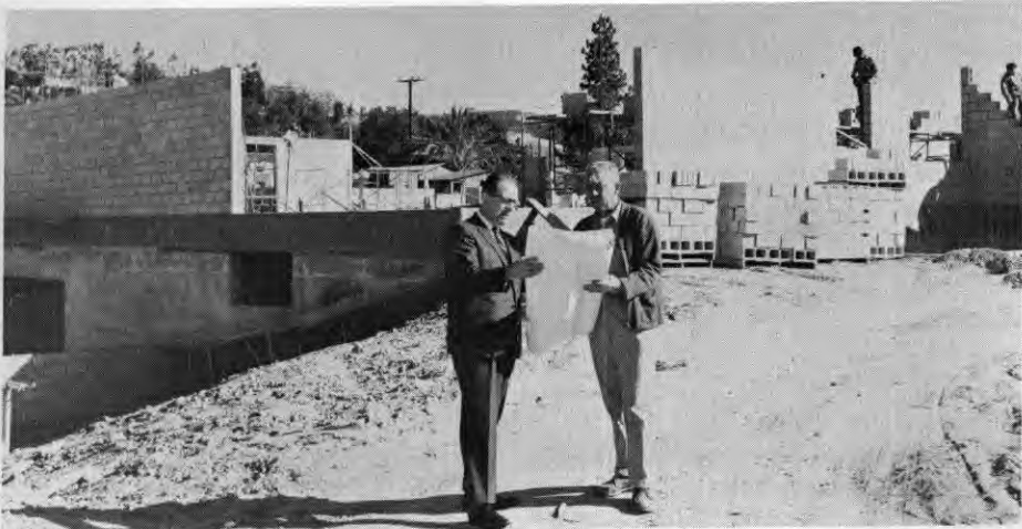
William H. Gosse (right), hospital administrator, and Arnold Steinert, construction superintendent, check over plans for the new Simi Valley Community Hospital which is under construction.
