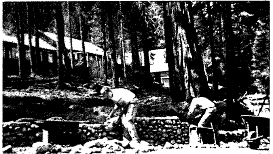
PROGRESS AT CAMP WAWONA.—Two fine young men, Don and Ervin Beasley, hard at work on the rock wall which will "dress up" the entrance to Camp Wawona.
