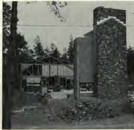
Looking east toward the kitchen and dining hall at the Prescott campground.
