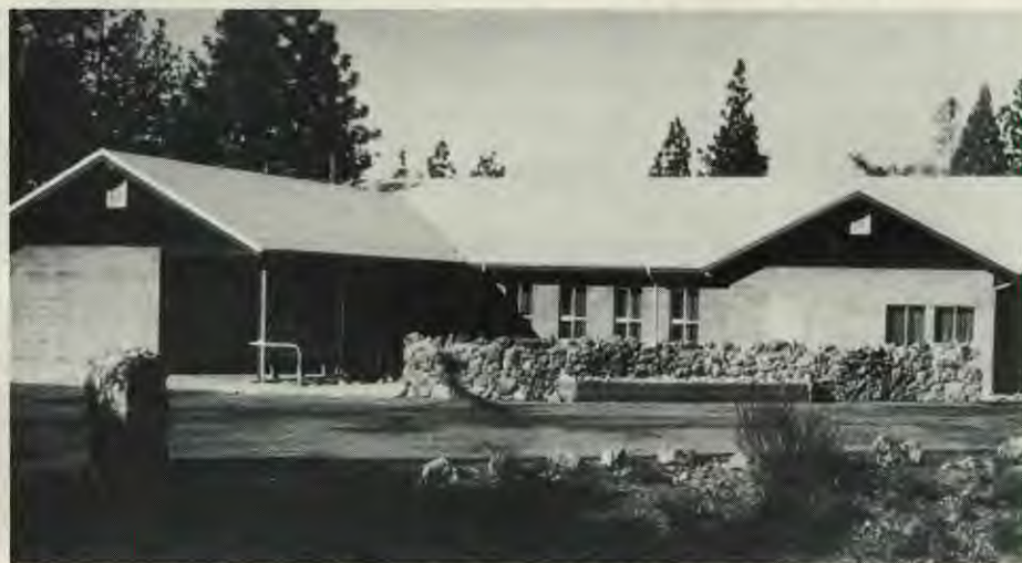
This new church at Colfax was dedicated in services held recently.
