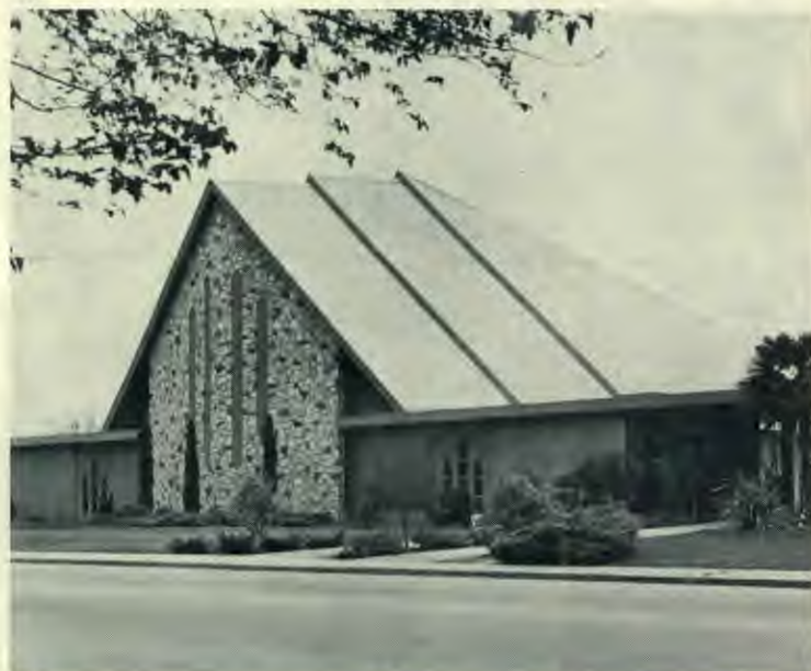
Visalia is planning church-dedication services May 16 and 17
