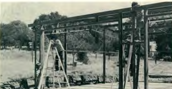
Pine Hills Junior Academy ninth- and 10th-grade boys are learning construction skills while building the new vocational arts structure.
