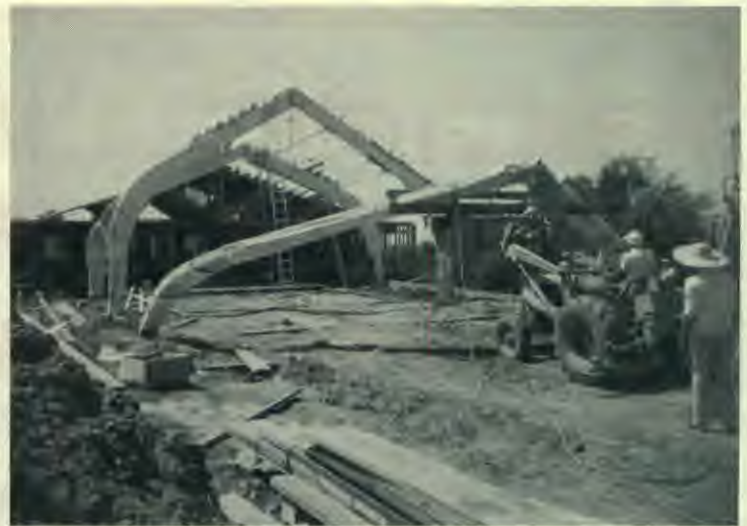
THE NORTH FORK CHURCH is growing. The last glued beam has been raised and the downstairs rooms have been enclosed. It is expected that the whole church will be closed in before the rains start.
