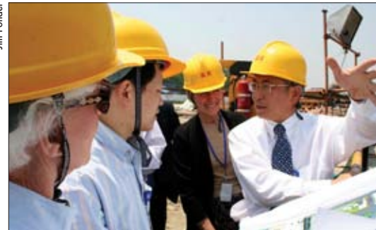
He Chao, M.D., right, president of SRRSH, reviews construction plans for the new 1,200-bed Xiasha Hospital with a delegation from LLU.
