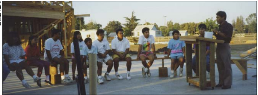
Volunteers gathered for vespers at the building site in September 1991.
