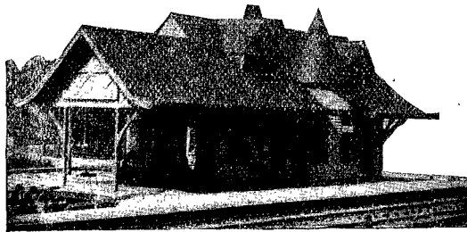
BALTIMORE &amp; OHIO RAILWAY STATION
