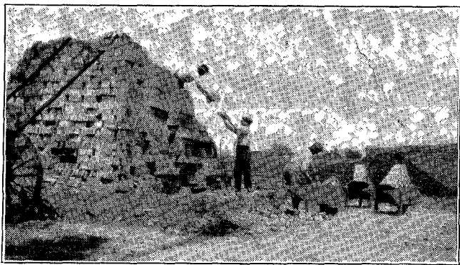
Unloading and piling bricks from first oven.
