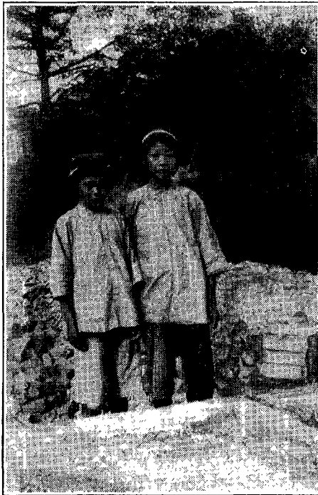
These two girls carried practically all the mortar for the new hospital building in China.
