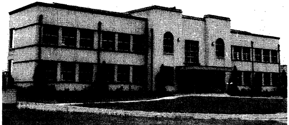
The administrative building of the new training institute recently established in Taipei, Taiwan (Formosa).
