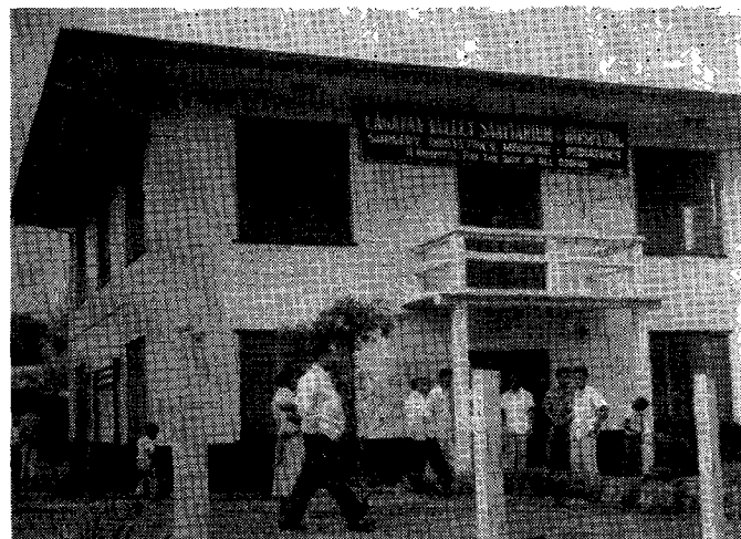
New hospital at Santiago, Isabela, Northern Luzon.
