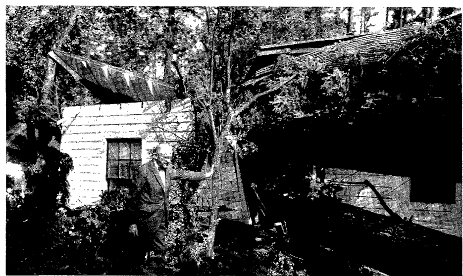
The Oregon Conference campground at Gladstone Park was damaged to the extent of $300,000 by the recent windstorm that swept up the Pacific Coast. Most of the damage was caused by falling trees. Top: H. L. Rudy, conference president, examines the damage to the camp office building. Center: Damage to one end of the primary division building. Bottom: Ruins of the teen-age pavilion.
