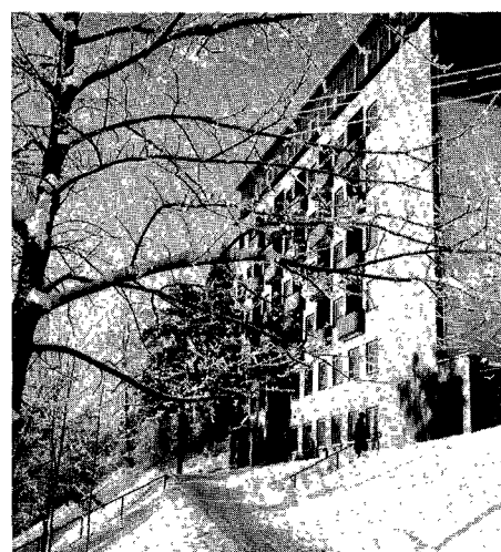
The recently completed new wing for the Hultafors Sanitarium, in Sweden, adds much-needed space for this institution.
