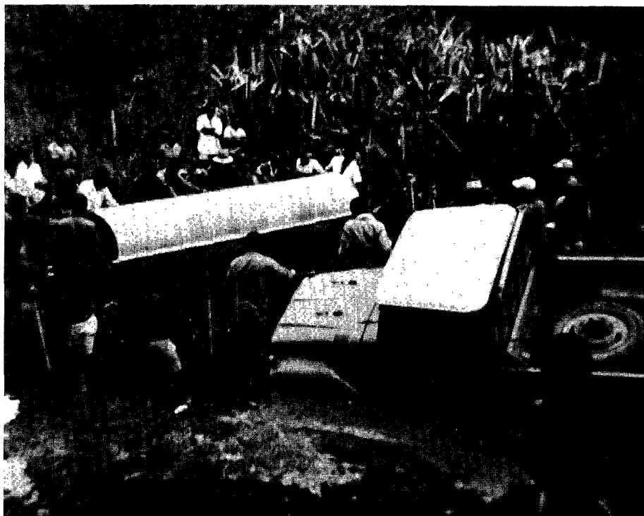
A typical plight on a New Guinea road. Drain pipes are being laid across the road.
