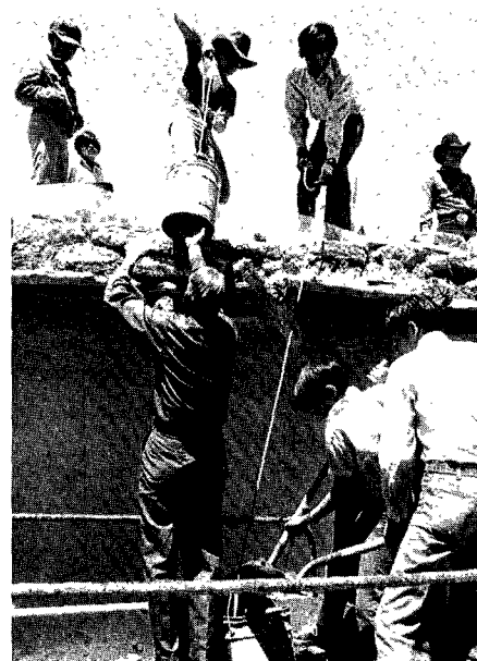
Left: Tayauoumana's house did not withstand this winter's unusually heavy rain. Top: Students brought in dirt to cover the plastic. Middle: Tayauoumana can now take down the plastic garbage-can liners that were tacked to catch the drips. Bottom: First step was to clear the top of the four-inch mud roof.
