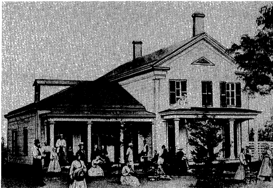
The Western Health Reform Institute, which opened in 1866 in an eight-room cottage, was the first Battle Creek Sanitarium building. The Seventh-day Adventist Church was instrumental in the opening of this hospital, although it never directly owned the institution.
