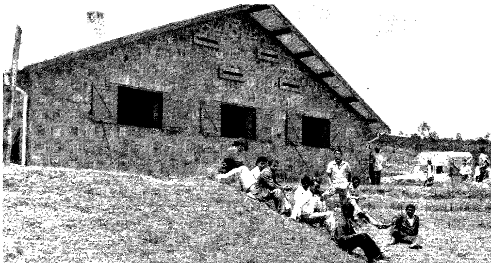
Three "chalets," a kitchen and dining lodge, bathrooms, and meeting facilities have been completed.
