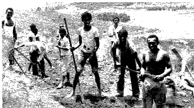
Madagascar youth are helping to build their new camping facilities.
