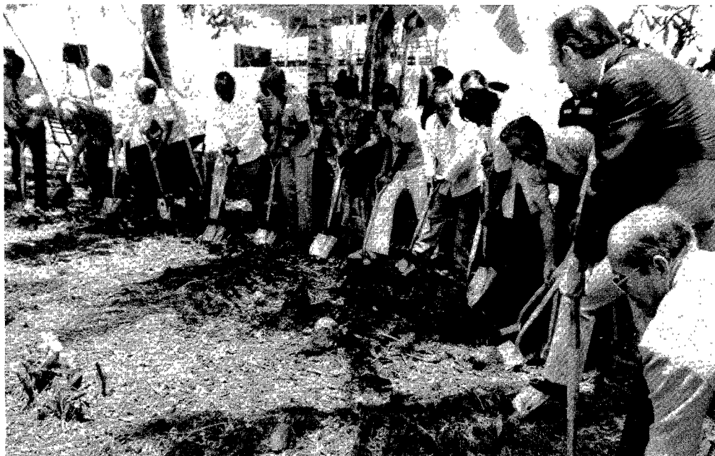
Sod-turning for the first new building at the new Silang campus of Philippine Union College symbolically inaugurates the move of the college from metropolitan Manila to its spacious rural location 45 miles south of the city.
