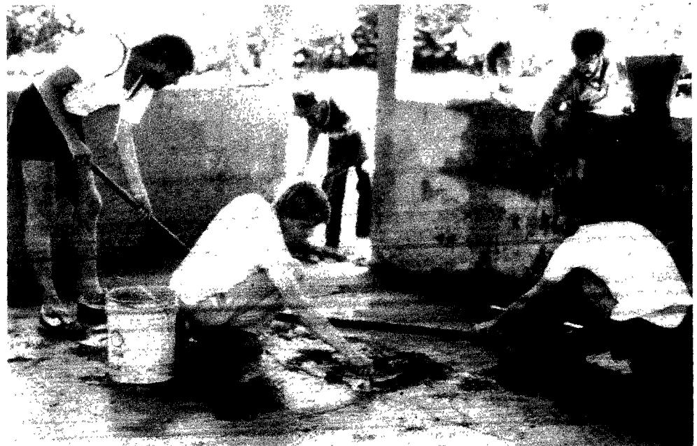
Loma Linda students helped finish the cement work on the schoolhouse at Clinica la Laguna.
