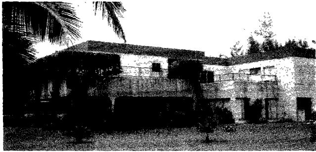
Working conditions should improve significantly for the staff of the Africa-Indian Ocean Division when they move out of their present cramped quarters into the recently purchased Indian Embassy (pictured above) in Abidjan, Ivory Coast.
