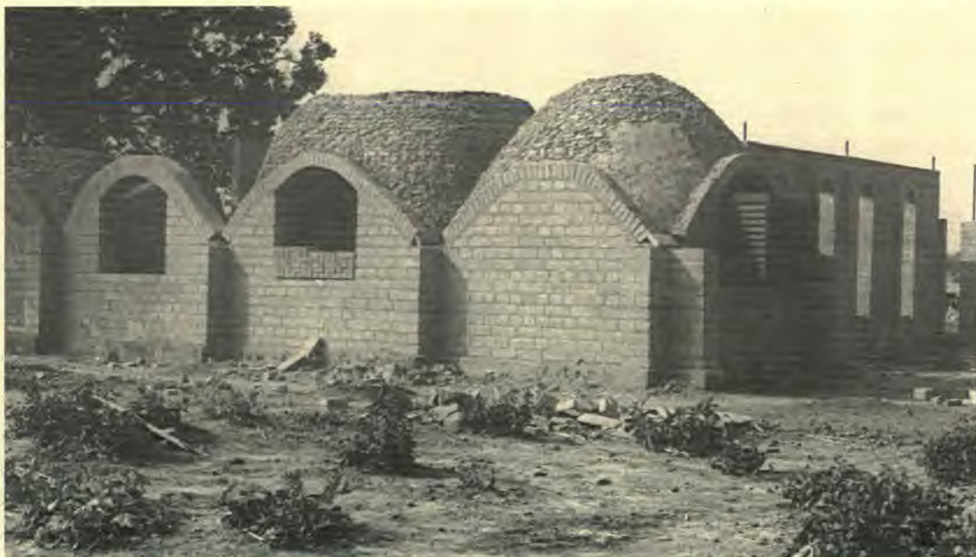
The unusual vaulted roof structure of the three ancillary halls is a traditional north African method of protecting the interior from equatorial heat. A thick layer of soil on top of the dome-like structures effectively insulates the building. The shade of the giant mango tree also helps. The section on the right is designed as a pharmacy for the district with a dispensing window on the right.
