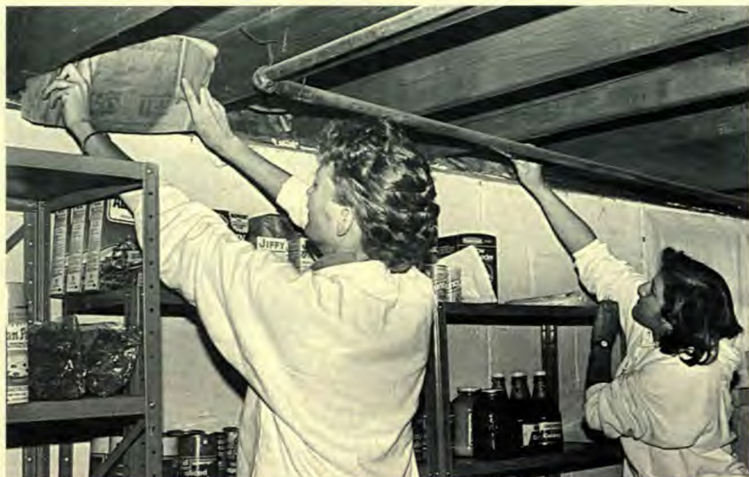
Left: Pam Sadler, Dave Sherman, and Nancy Steely cut the fiberglass to be used for installation in one of the "bundle up blitz" homes. Right: Patti Wilson-Short and Pam Sadler fit fiberglass against the outer walls to protect from cold outside air.
