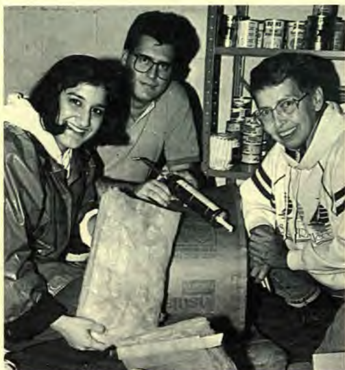
Left: Pam Sadler, Dave Sherman, and Nancy Steely cut the fiberglass to be used for installation in one of the "bundle up blitz" homes. Right: Patti Wilson-Short and Pam Sadler fit fiberglass against the outer walls to protect from cold outside air.
