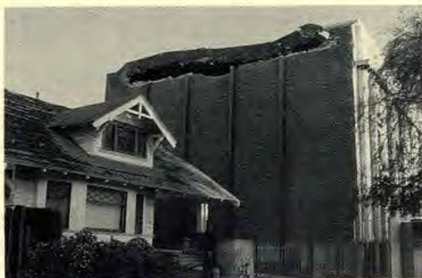
The University church incurred extensive roof damage.
