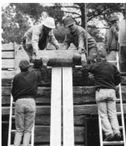
BRICK BY BRICK: Just kidding. There're no bricks in this log cabin. However, the two-story structure had to be taken apart at its original site, moved to the village, and reassembled.
