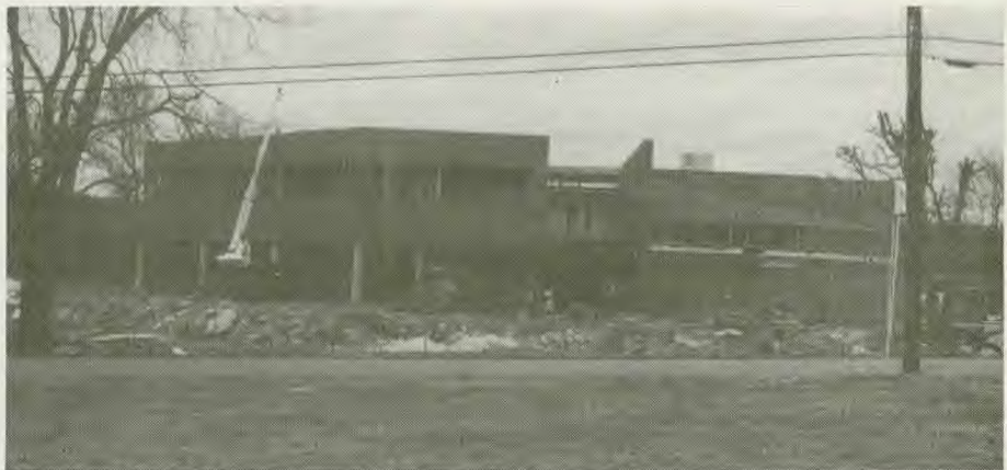
South Central Conference office building nears completion.
