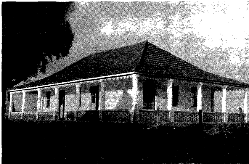
Building in which Classes are Conducted.
