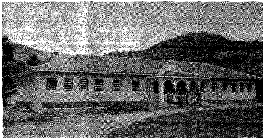
Administration Building Northeast Brazil Academy.
