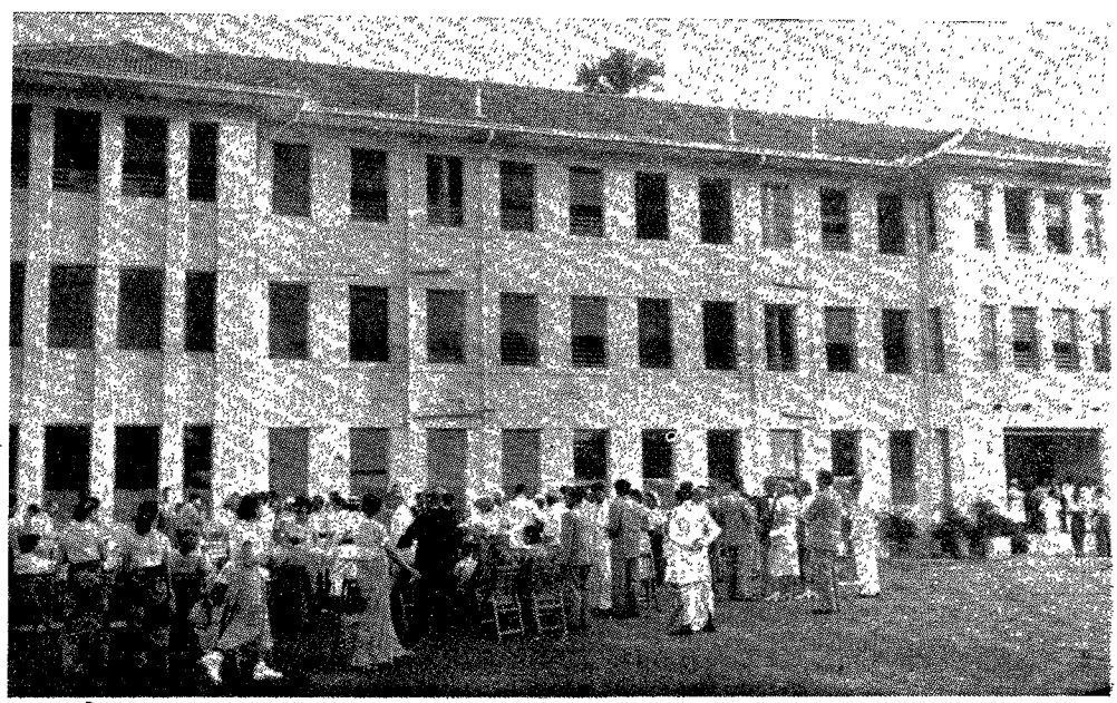
The new wing of the Seventh-day Adventist Hospital, Rangoon, Burma, which was opened on January 2, 1955.
