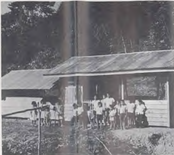
INNOVATION. The very first lamb shelter in the Far Eastern Division was built in Togop, Sabah. This is how it looked on the day of its dedication in March of 1967.
